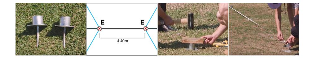
Use the supplied triangle peg placement template mark out the position of each peg. It's important that the template steps(Figure 02) to follow to identify correct peg placement, failed to follow these steps will result in your marquee not sitting in the correct position and may cause damage to the marquee.
